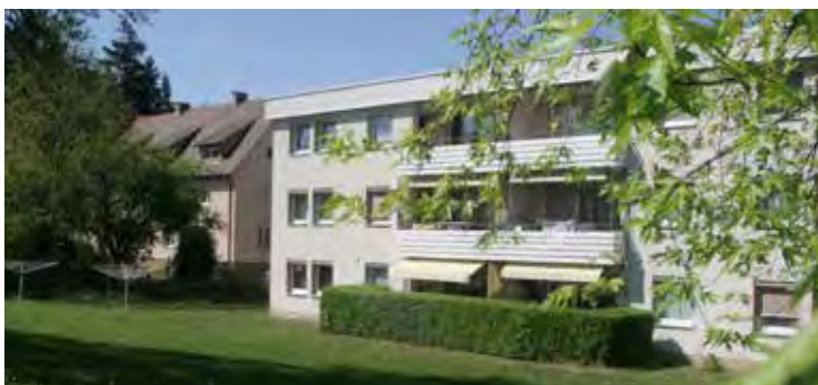
links: Neue-Wolterdinger-Straße 19 . rechts: Neue-Wolterdinger-Straße 17
